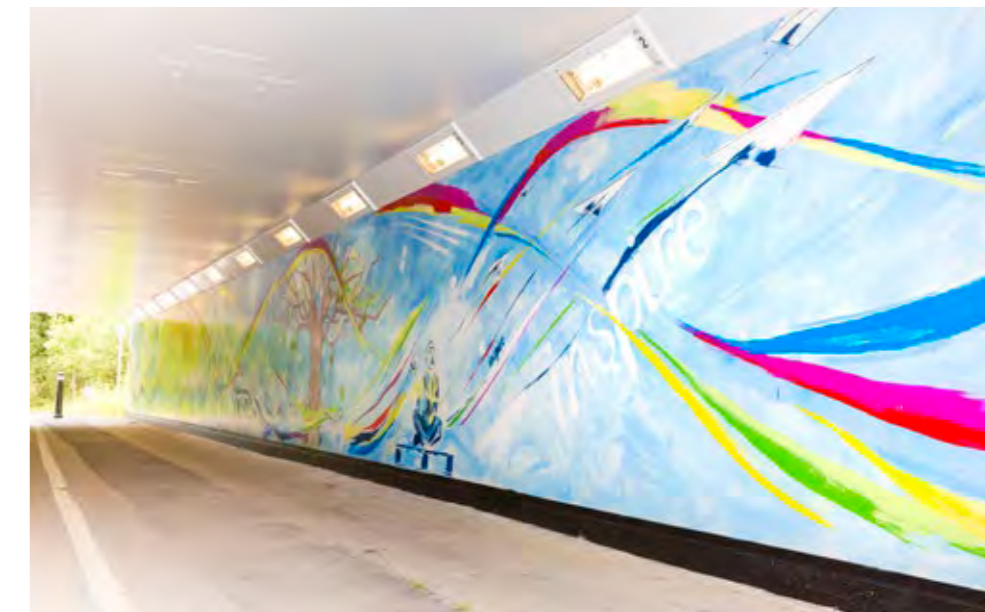
Green Lane subway
