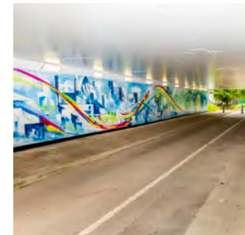
3. Green Lane subway
