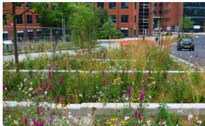
Rain gardens take the surface water run off, add character and provide opportunities for biodiversity. They can also change throughout the year.
