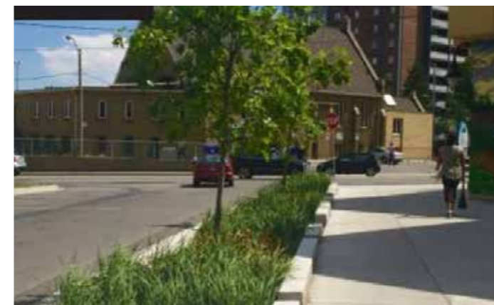
Hit and miss kerbs enable surface water from hard surfacing to fall into swales and rain gardens.
