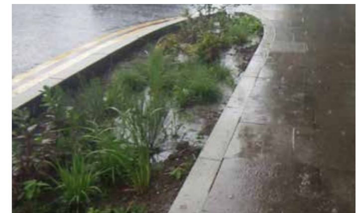
Rain water conveys into rain gardens close to where it falls. The rain gardens act like sponges whilst providing amenity and biodiversity to the public realm.
