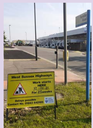
WSCC repairing pavements
