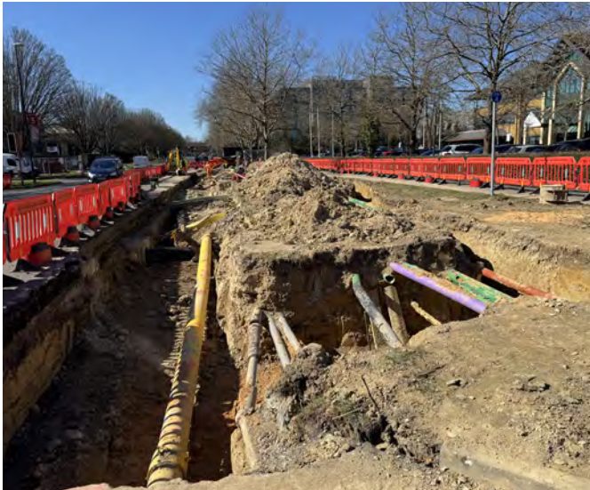
Image of Manor Royal Road showing complexity of underground services beneath existing grass verges.
